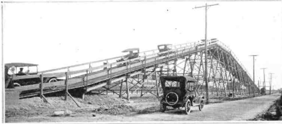
Dodge Bros., Detroit, Mich., have completed a 1/2-mile speedway, test hill and sand pit on the factory grounds for the purpose of testing their test men off the public streets and roads. The hill is 532 ft. long by 39 ft. wide and has two approaches with varying grades. Over 215,000 ft. of lumber is used in the track, in which no pedestrians are allowed.
